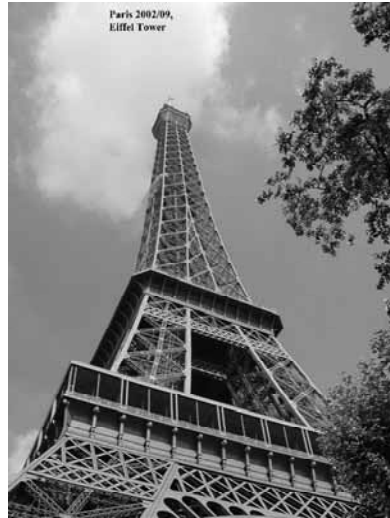
Architectural Structures I ENDS 231
