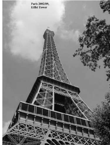
Architectural Structures I ENDS 231
