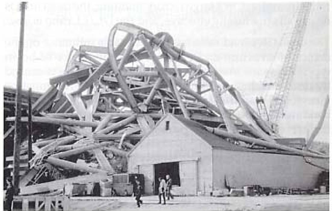
Figure 1.15 Stability and the strength of a structure—the collapse of a portion of the UW Husky stadium during construction (1987) due to a lack of adequate bracing to ensure stability. Photo by author.
