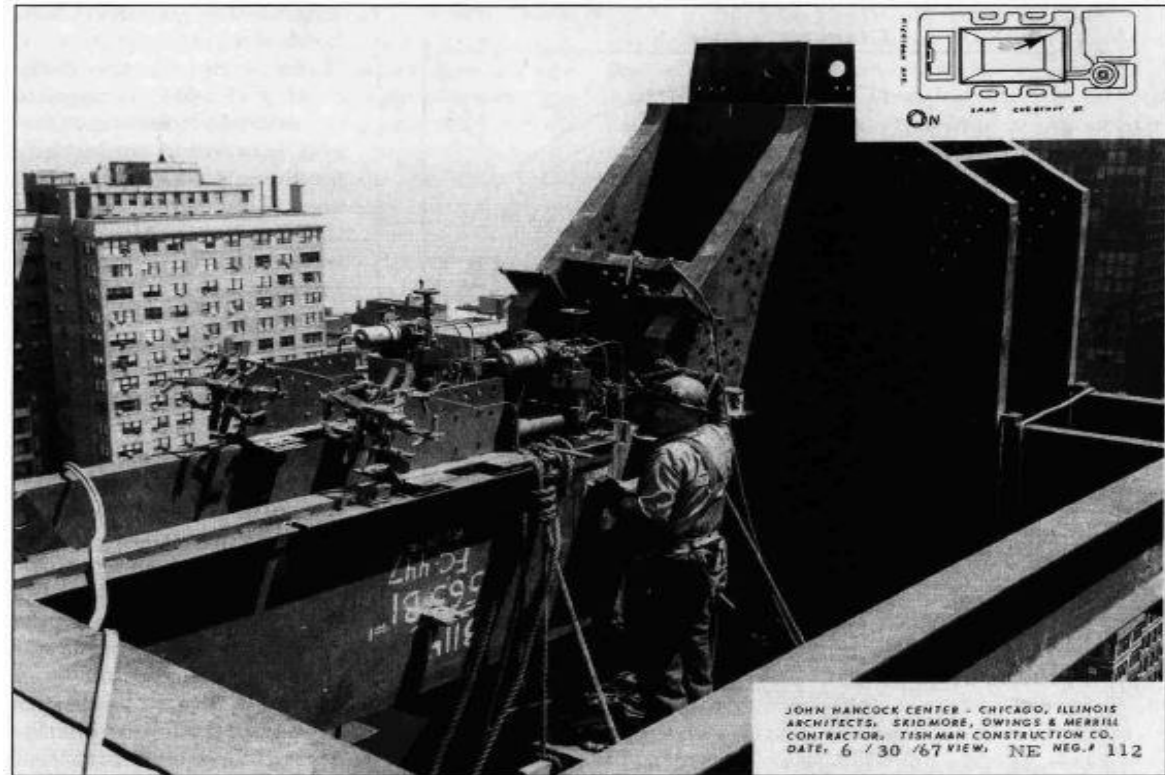
This construction photo reveals the scale of the prefabricated main joints. (Courtesy of Skidmore, Owings & Merrill LLP.)
