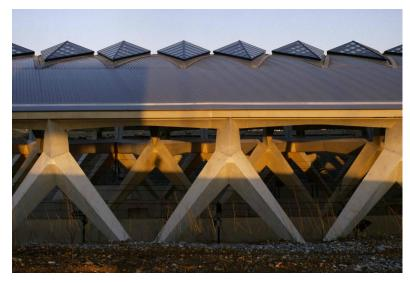
• Because of the density of the concrete beam network and its longitudinal character, the railway cover resembles a tunnel lit by natural light.
