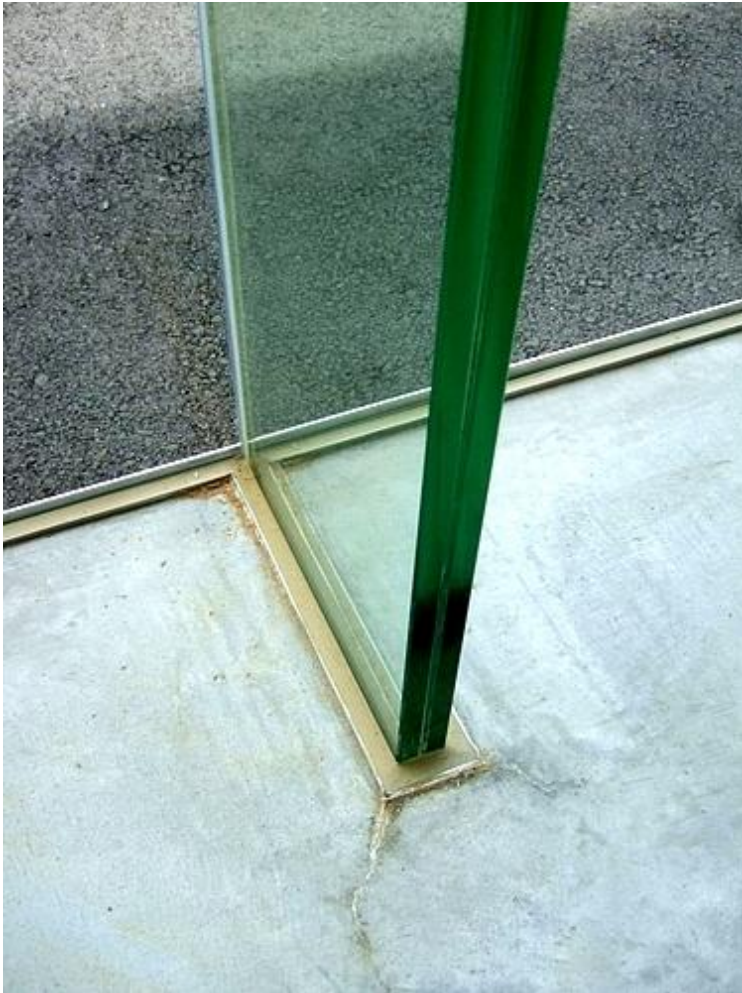
Glass wall are around. Installing a glass rib helps it stability.
