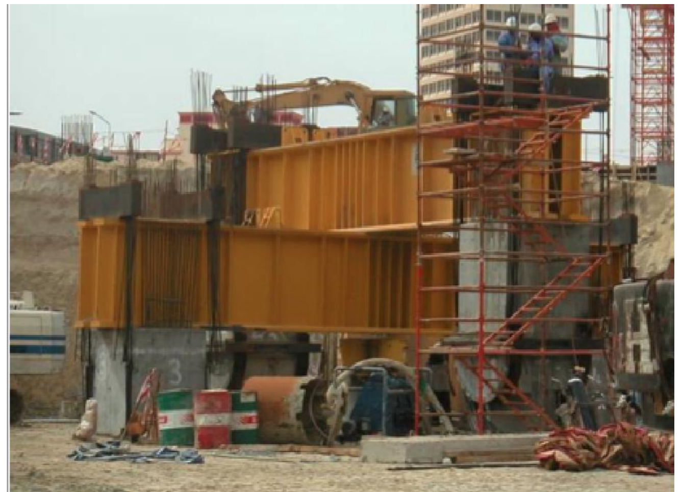
ON SITE PILE LOAD TESTING
