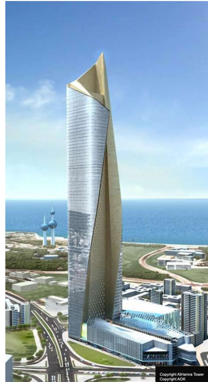
★ AL HAMRA TOWER, KUWAIT CITY
