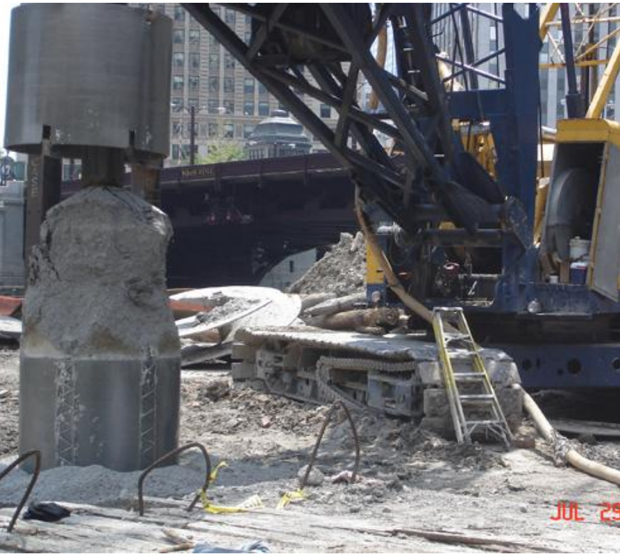
Rock is reduced to sand and gravel by downhole hammer tool .
