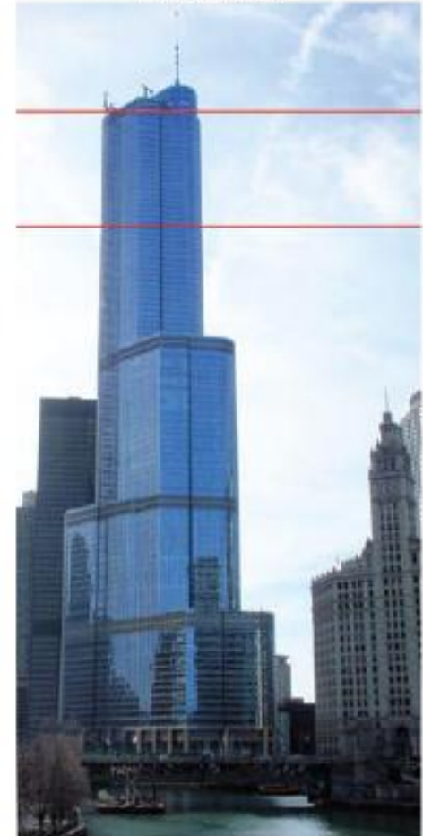
PHASE 5 COMPLETE AND OCCUPIED (HIGH RISE CONDOS) MAY, 2009
