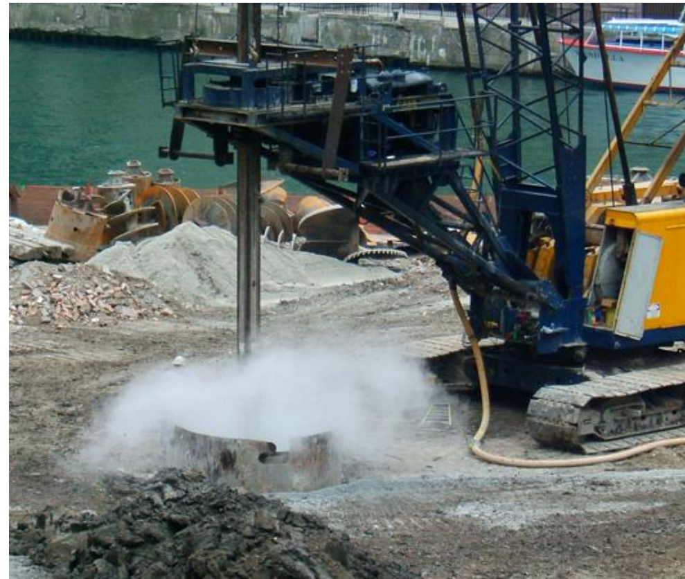
Rock socket drilling with air-operated downhole hammer tool
