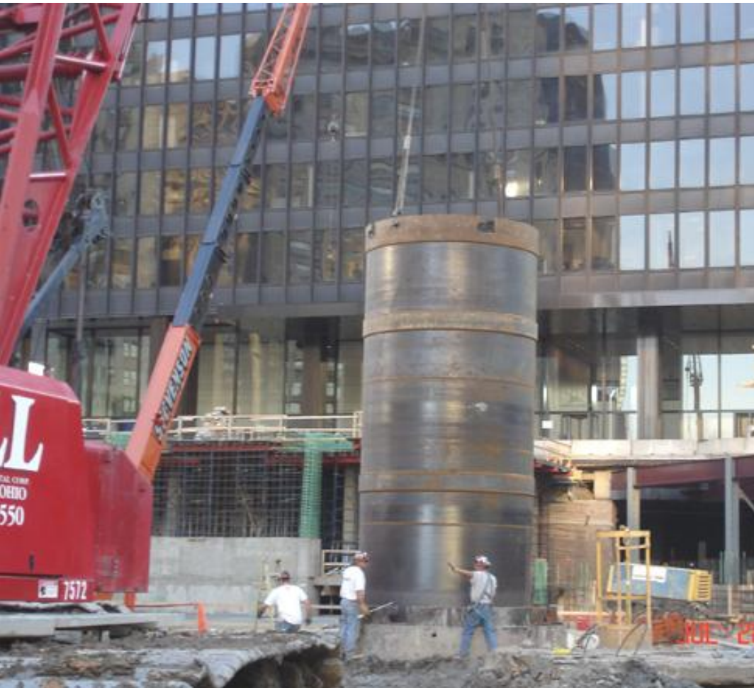
Installation of 10ft diameter permanent casing for Tower rock caisson
