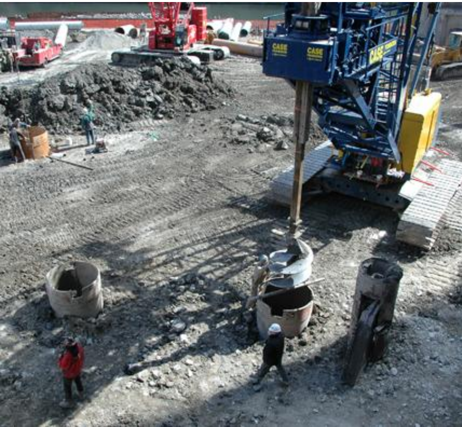
Large crane attachment drill augering 8ft diameter caisson shaft to rock
