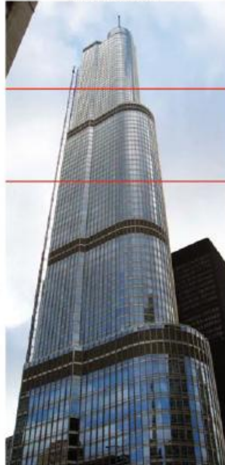
PHASE 4 COMPLETE AND OCCUPIED (MID RISE CONDOS) MAR, 2009
