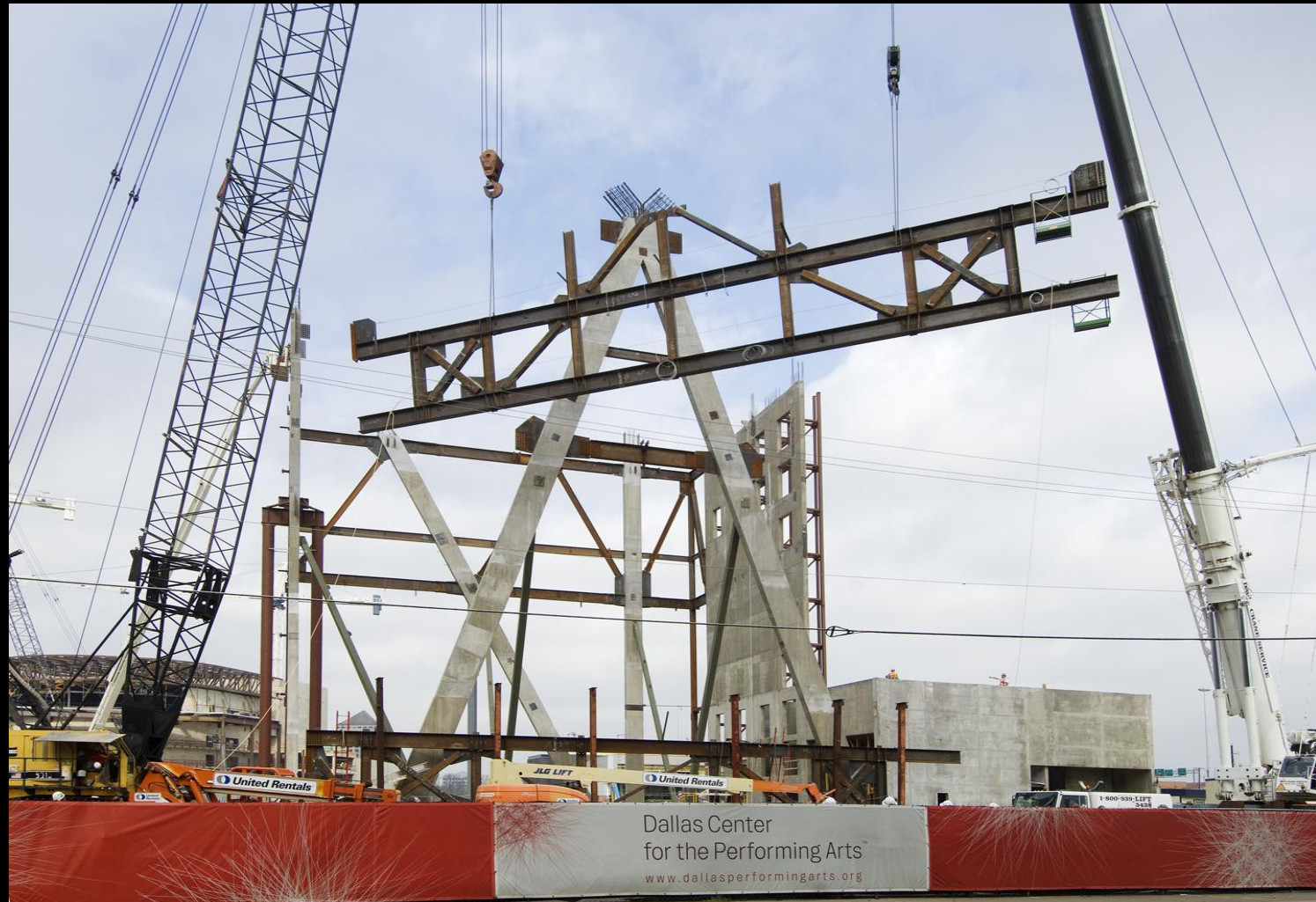
T2 Truss being lifted over 92' Columns
