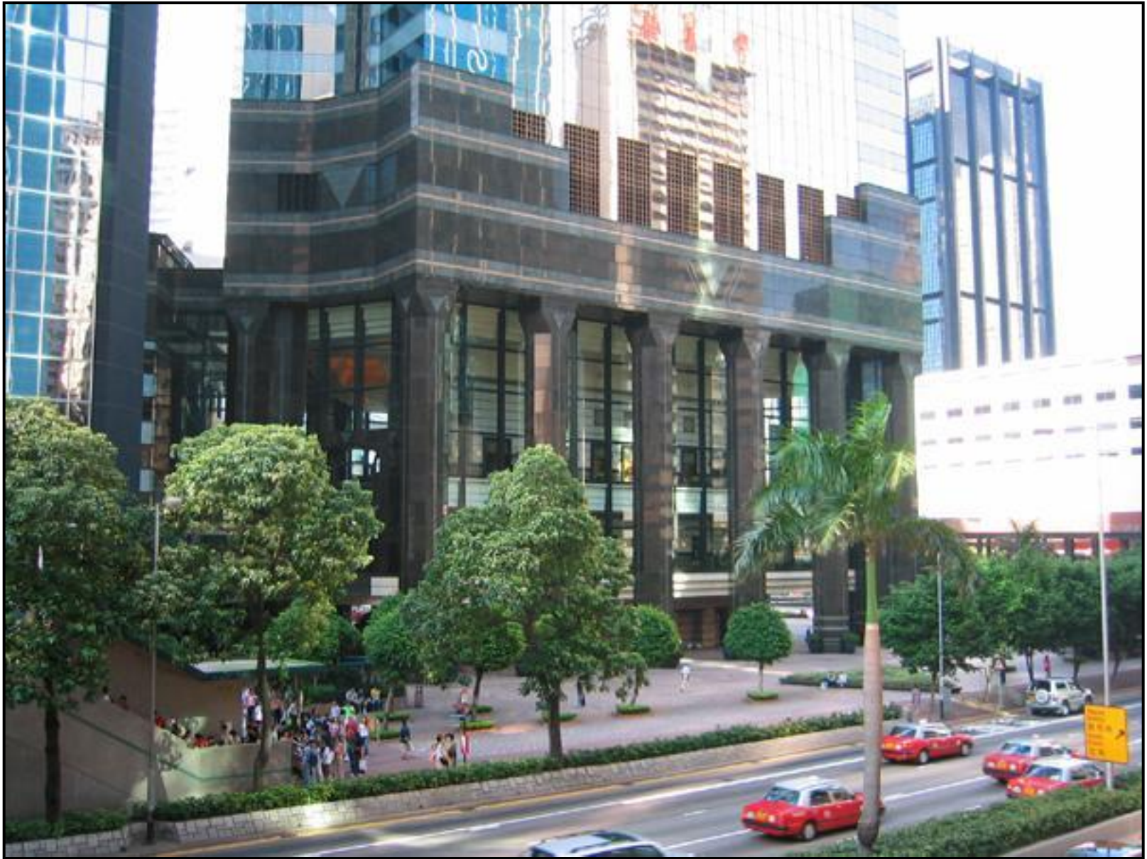
THE ENTRANCE PODIUM -30.5 M HIGH with 2m dia and 8.6 m spacing of concrete columns M60 grade
