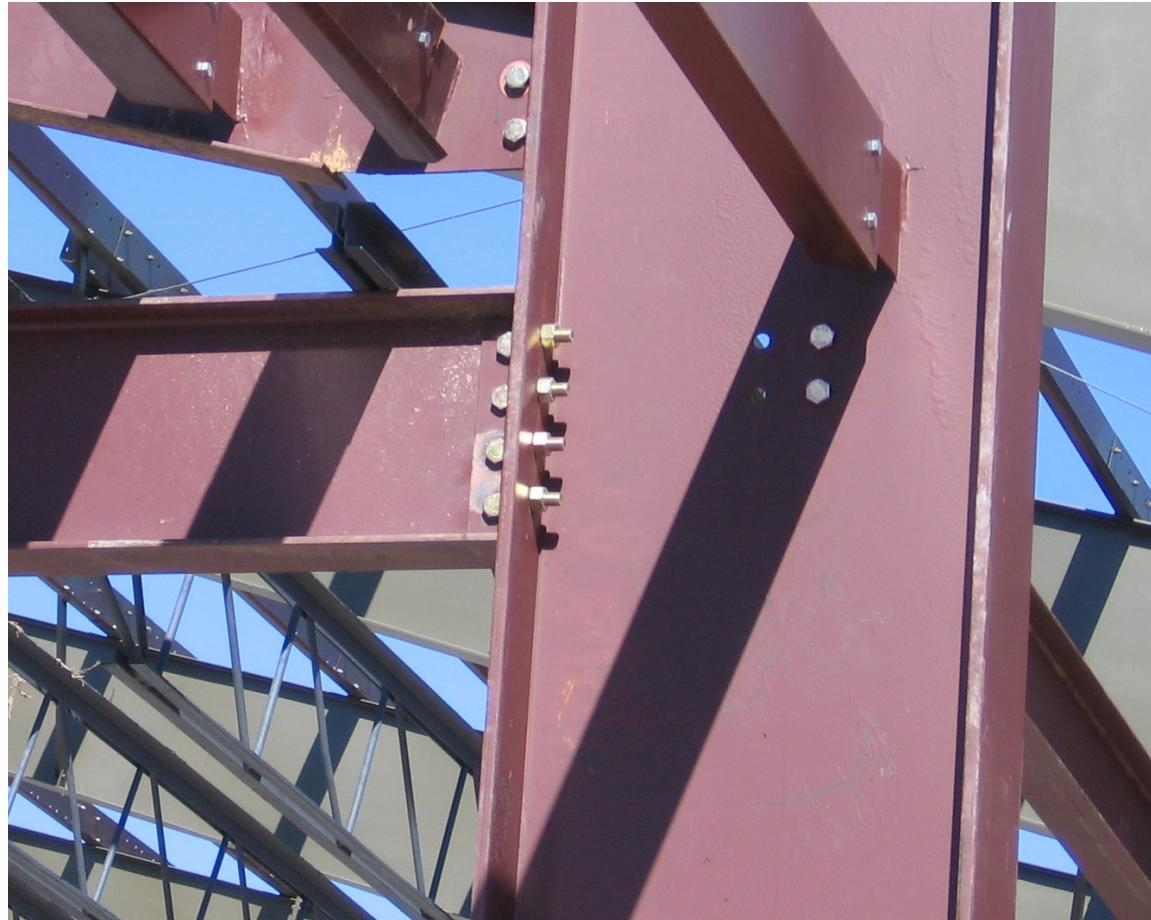
The bolts hold the beam in place for welding and also provide shear resistance. Groove welds develop the full strength of the flanges of the beam.
