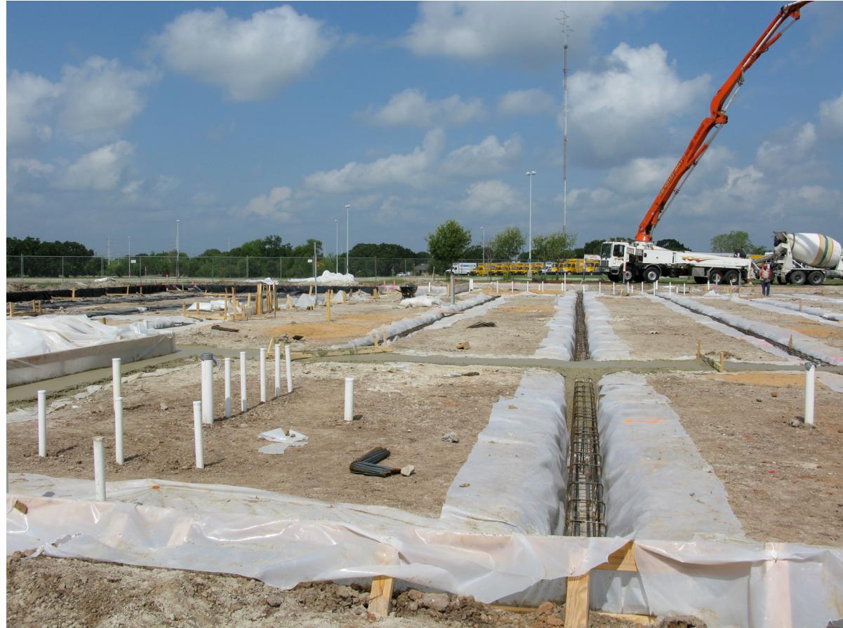
The foundation system for the building is a two-way slab with grade beams supported by piers. The foundation accepts the concentrated loads of the building and spreads them over a large area of soil. Several different parts of the foundation, i.e. the piers, footings, and grade beams, help transfer the loads.
