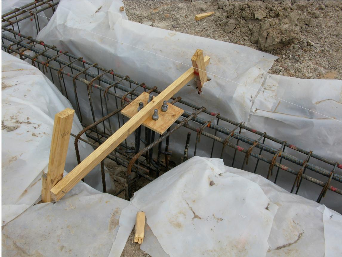
The grade beams transmit loads from bearing walls into spaced foundation, as the pier shown in this photo.
