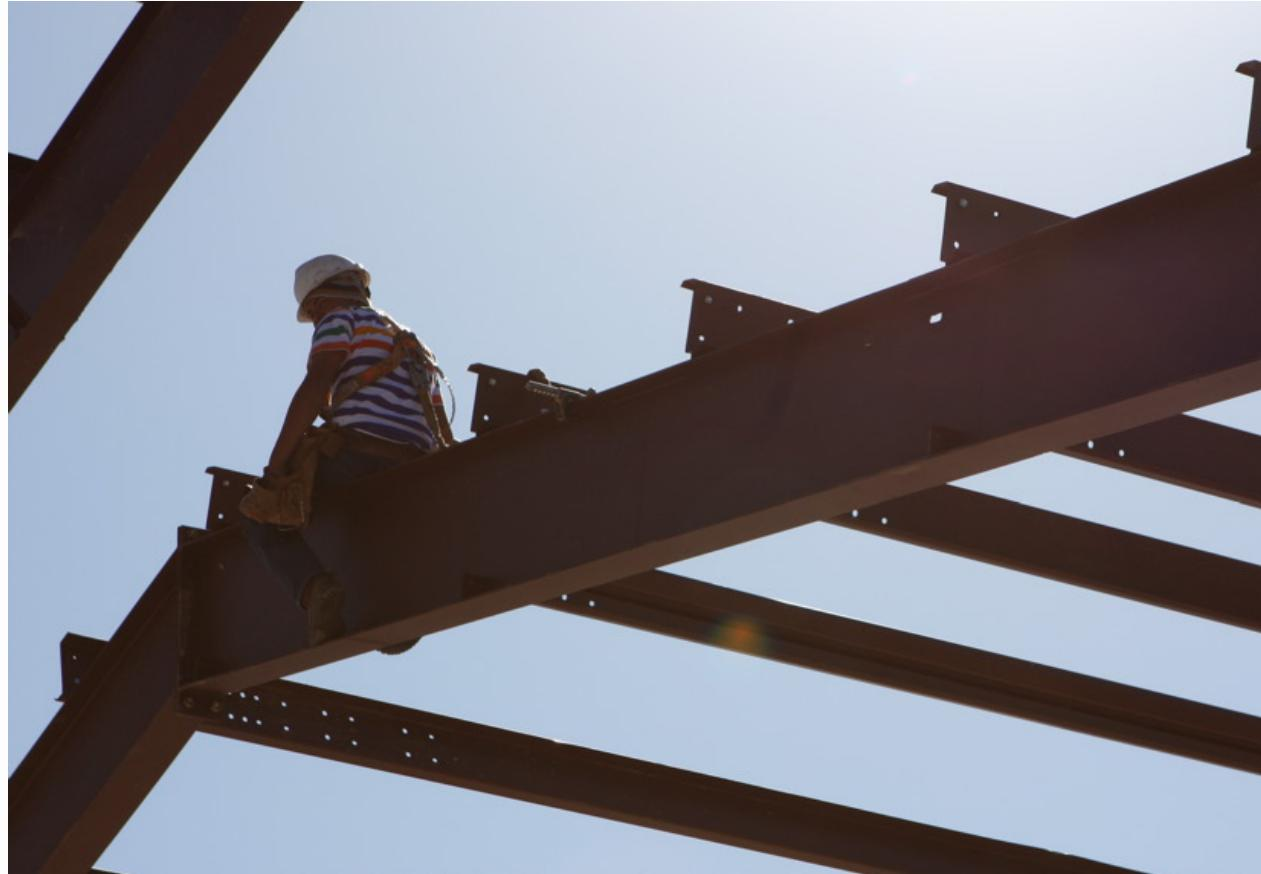
Steel purlins run horizontally between the steel rigid frames and support the roof deck as well as providing lateral support.
