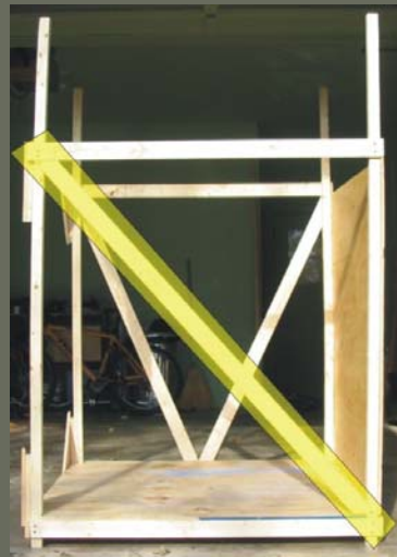
Diagonal Cross Bracing
