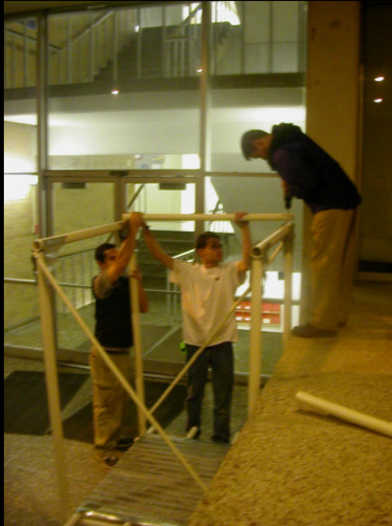
Josh, Steve and Bryan attach those stabilizing beams.
