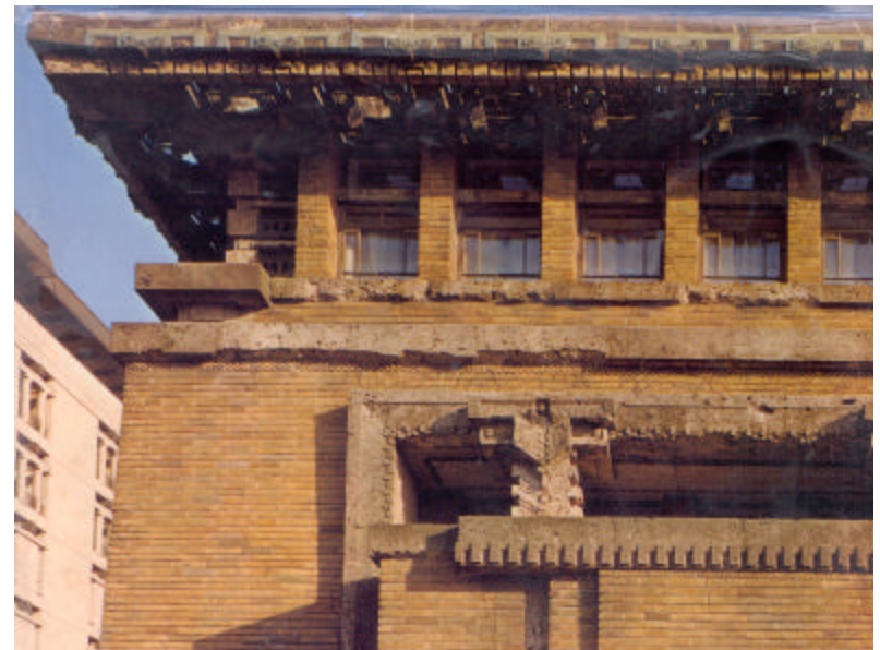
Detail of exterior wall and brick
