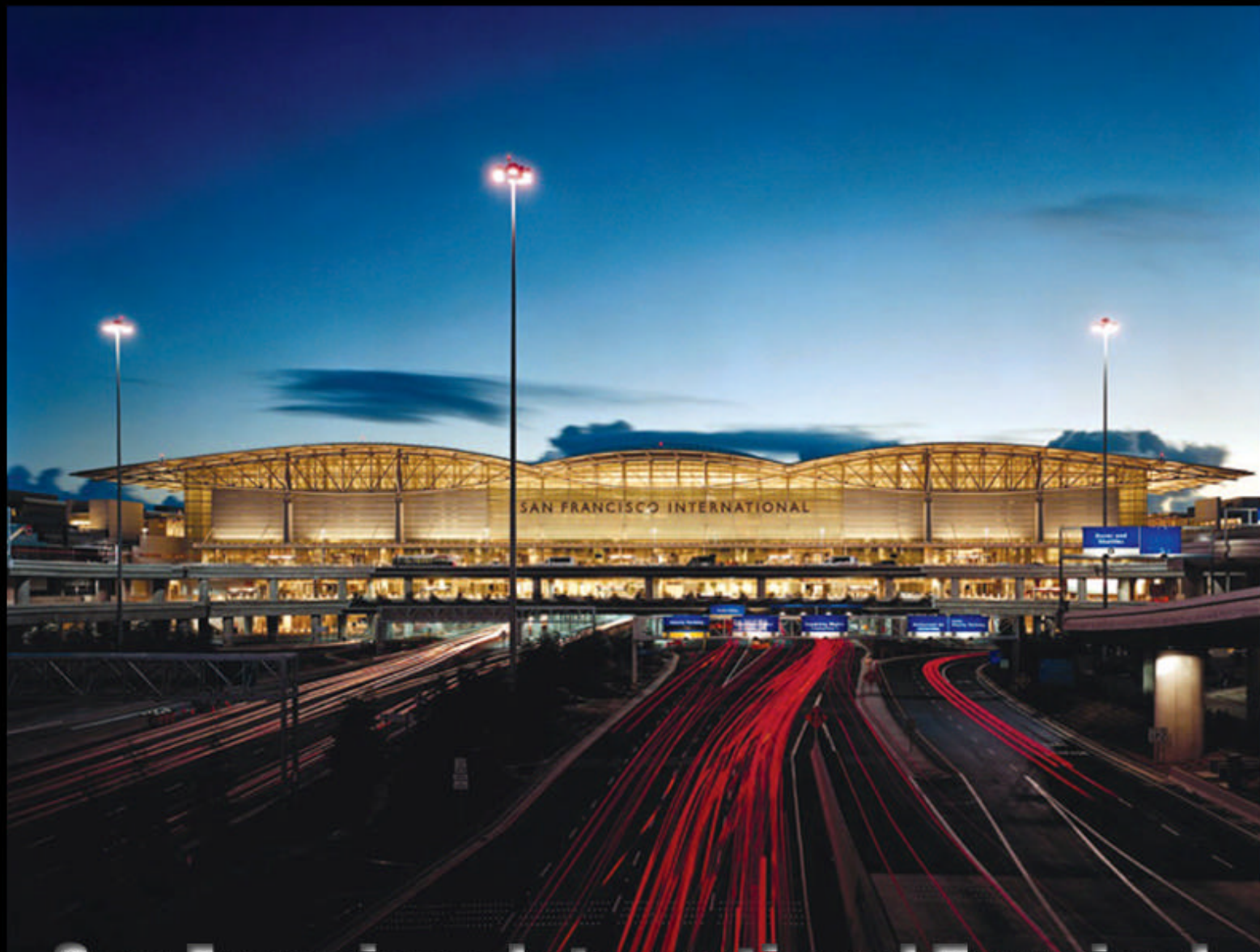
San Francisco International Terminal, San Francisco, California.
