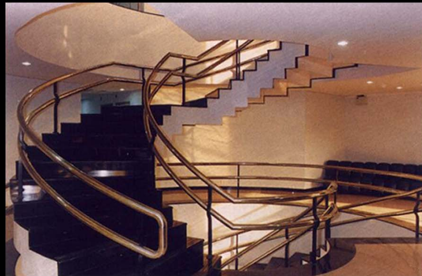
RCC HELICAL STAIRCASE
