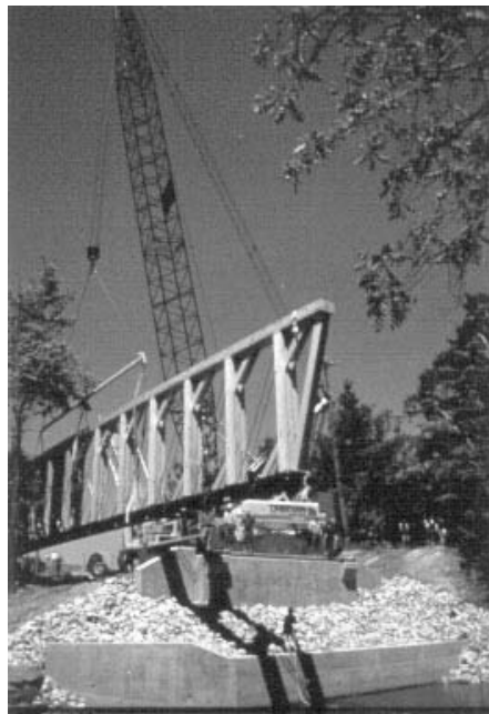
Glued laminated timber truss.
