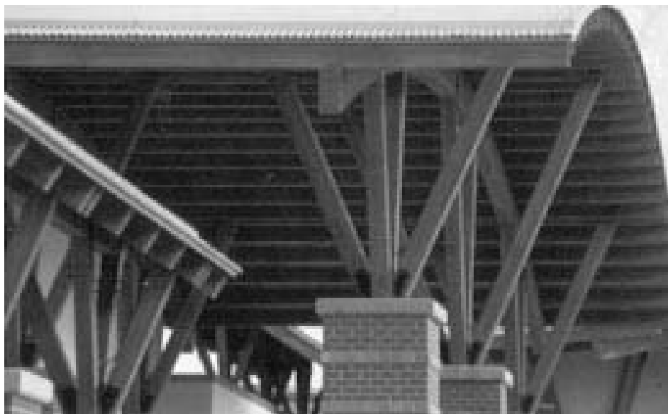
Grant Creek Shopping Mall, Missoula, MT; Architect--Fehlman-Labarre Architects; Contractor--Quality Construction
