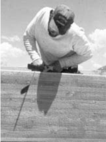
Field cutting a stock beam.
