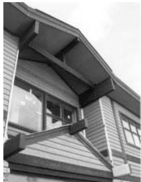
Office Building Remodel, Jackson, WY.
