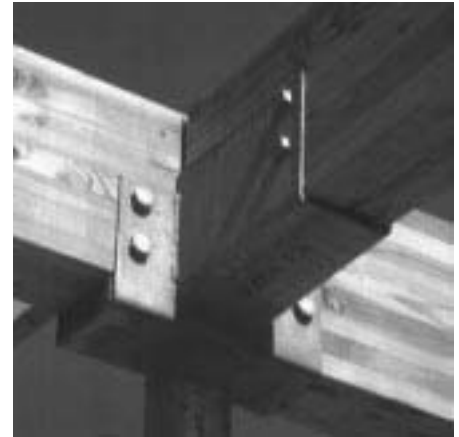
Beam Intersection connection.
