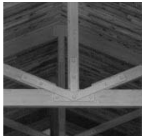
Truss connection.
