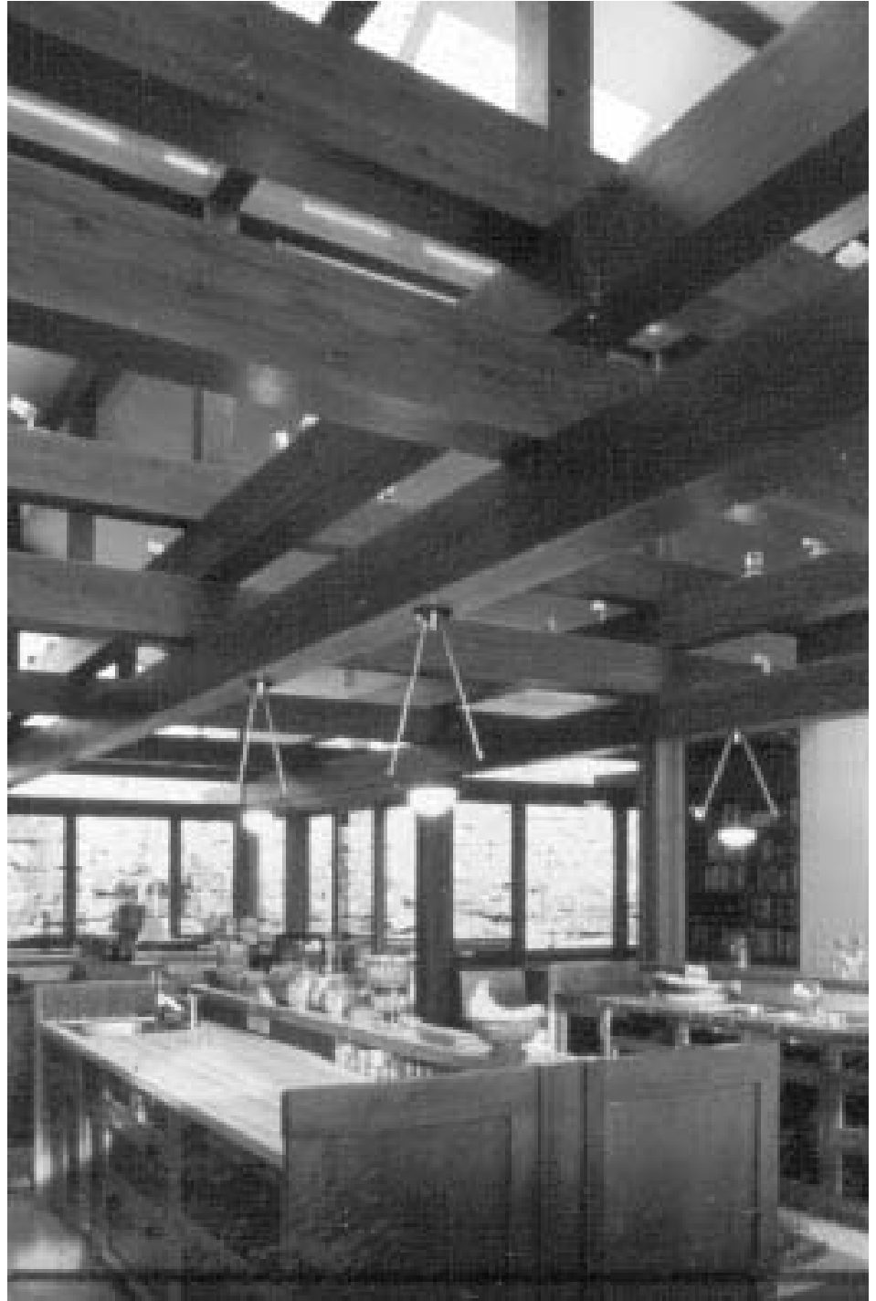
Sun Valley, ID Residence; Architect—Jack Smith, F.A.I.A.; Structural Engineer—Purdy and Associates; Contractor—Premier Construction Company.
