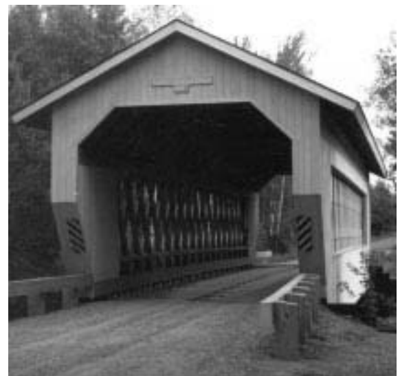
New covered bridge with laminated trusses; Engineer—USDA Forest Service.
