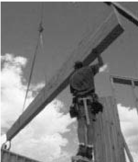
Installing a residential ridge beam.
