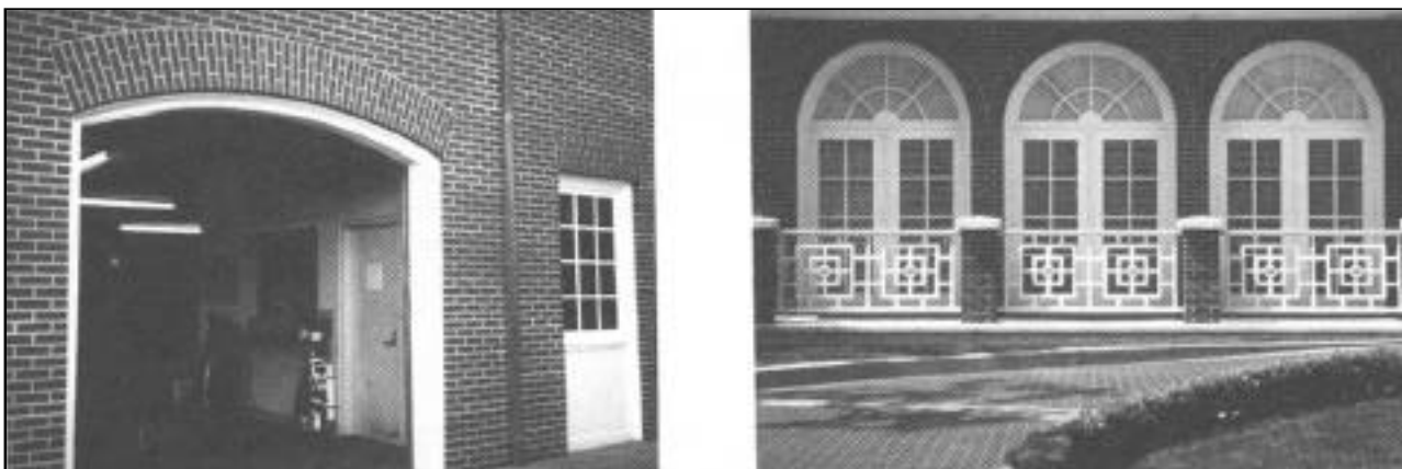
Structural Brick Arches FIG. 1
