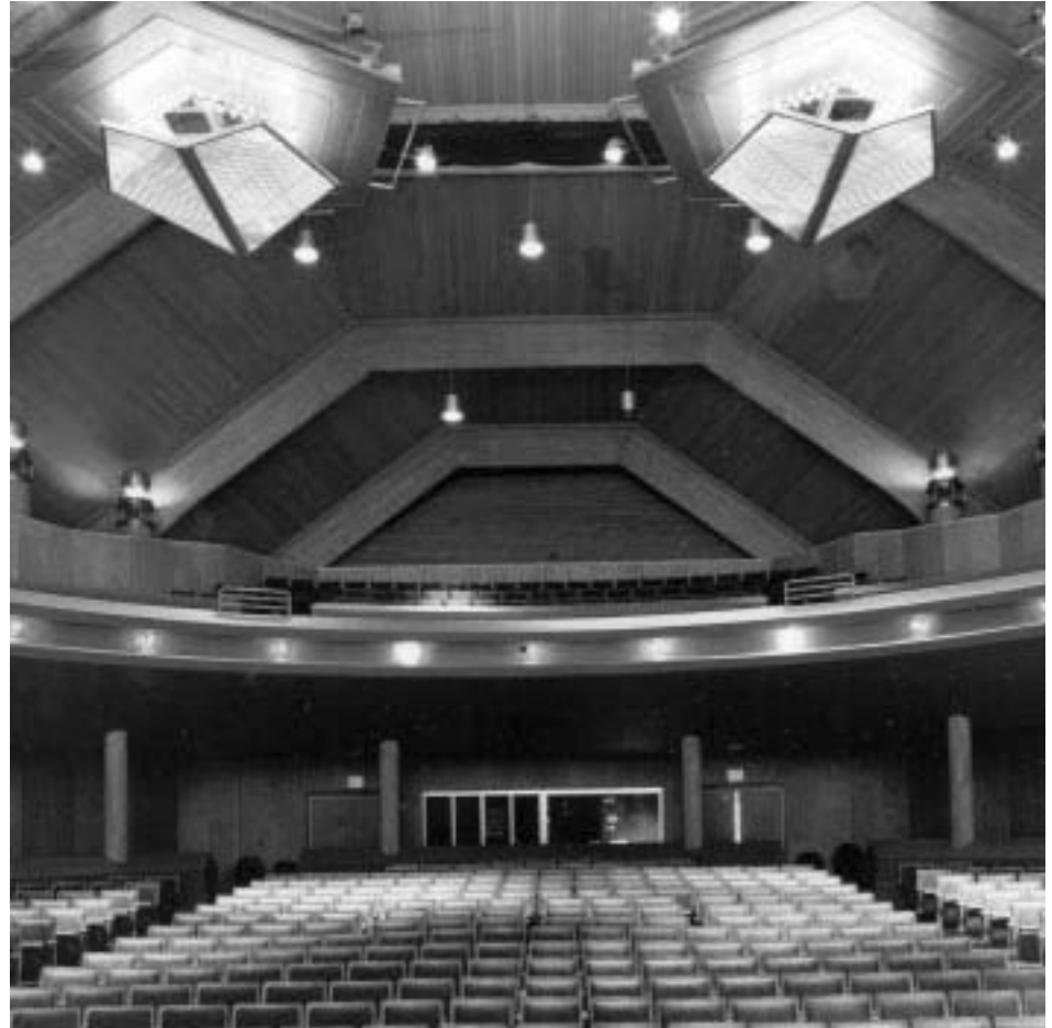
Wood ceilings and beams were selected for acoustical control. Performing Arts Center, North Texas University, Denton, TX; Architect—KVG Gideon Toll Architects; Engineer—Freese and Nichols, Inc.; Contractor—Huber, Hunt and Nichols, Inc.
