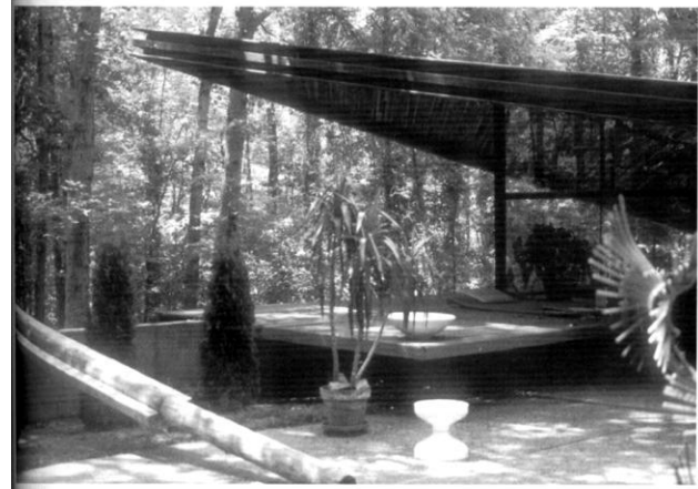
Figure 8.261 Residence with hyperbolic paraboloid roof, showing the ample overhang of the roof, the boundary members, and columns in the glass walls.
