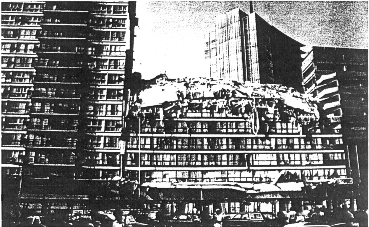
Figure 2.5: Building adjacencies can have major impacts on performance during earthquakes. A large number of structures suffered pounding damage during the 1985 Mexico City event, leading in many cases to partial or full collapse.
