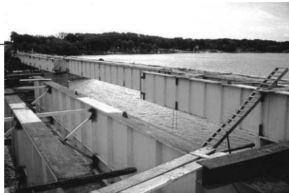
stiffeners at end where shear is greatest and at support
