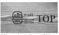
AITC mark of quality. The word "TOP" identifies beams with unbalanced sections.
