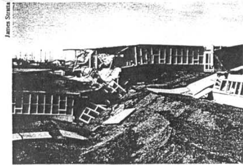
Figure 1.3: School straddling a landslide-induced rupture, Alaska
