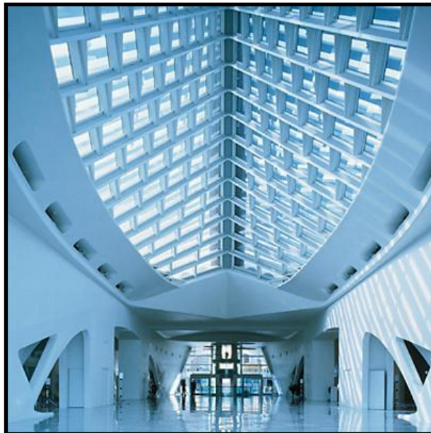
Figure 8: Pavilion Ring Beam (perimeter) and A-frames
