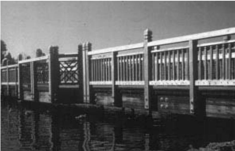
Bridge in Nature Park, Portland, OR, pressure treated with environmentally friendly copper naphthenate. Structural Engineer—Ceccacci Associates.
