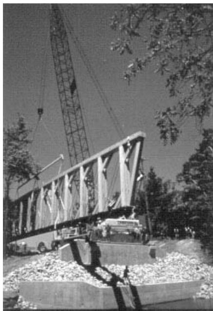
*Glued laminated timber truss.*
