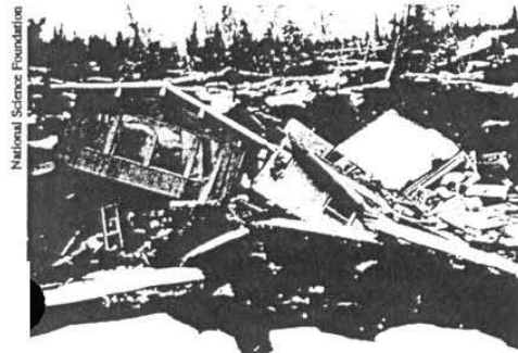
Figure 1.4: House on Turnagain slide
