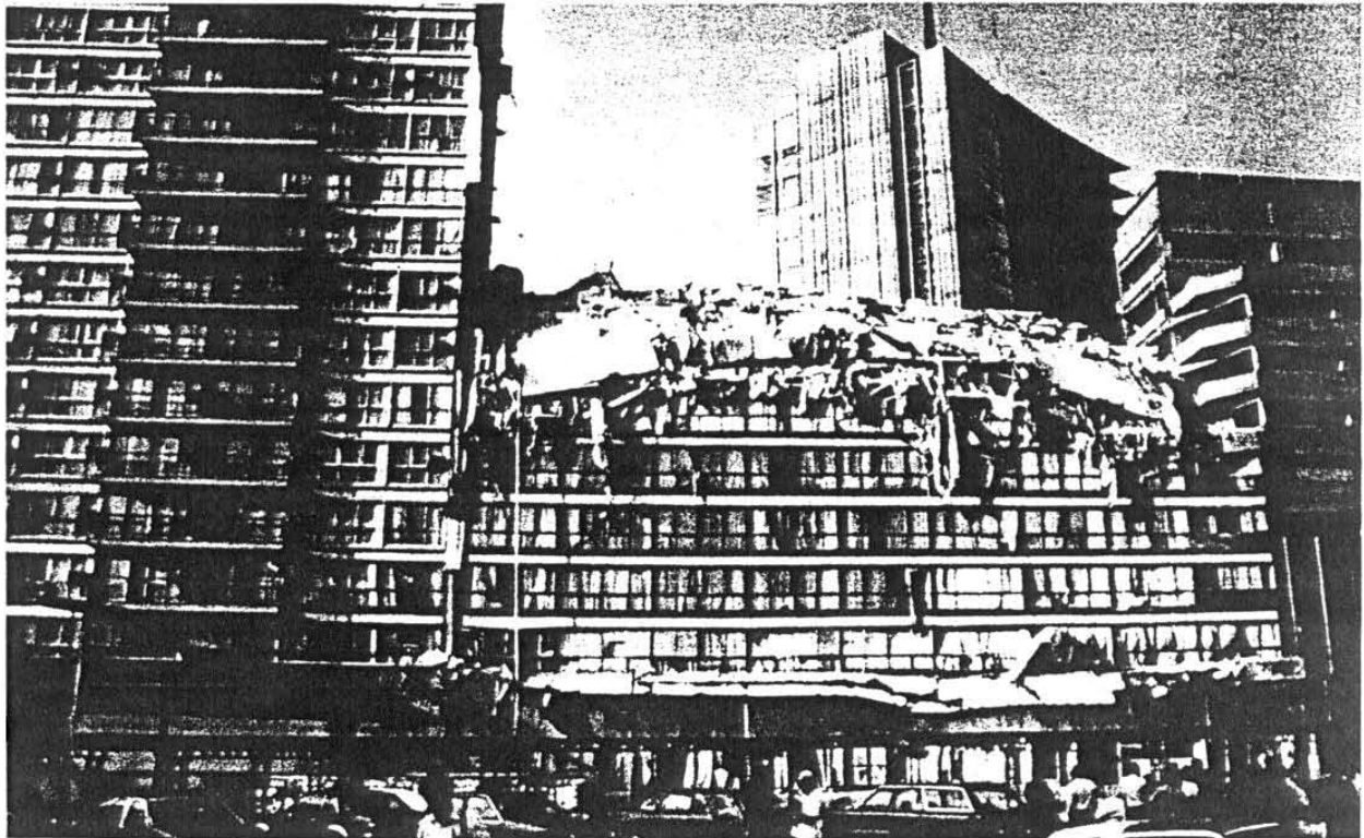
Figure 2.5: Building adjacencies can have major impacts on performance during earthquakes. A large number of structures suffered pounding damage during the 1985 Mexico City event, leading in many cases to partial or full collapse.
