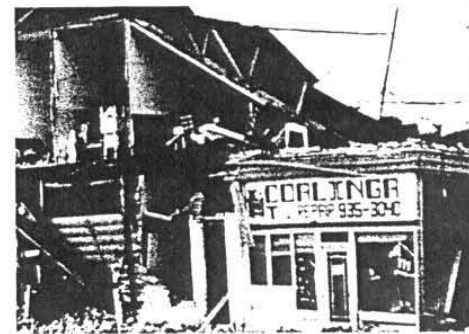
Figure 1.12: Damage to an older masonry building
