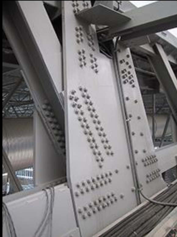
(AISC - Steel Structures of the Everyday)
