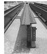
(AISC - Steel Structures of the Everyday)
