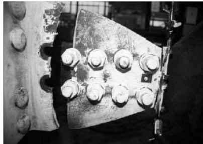
Figure 2-14. Tension Fracture Limit State (Photo by J.A. Swanson and R. Leon, courtesy of Georgia Institute of Technology)
