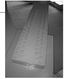
(AISC - Steel Structures of the Everyday)
