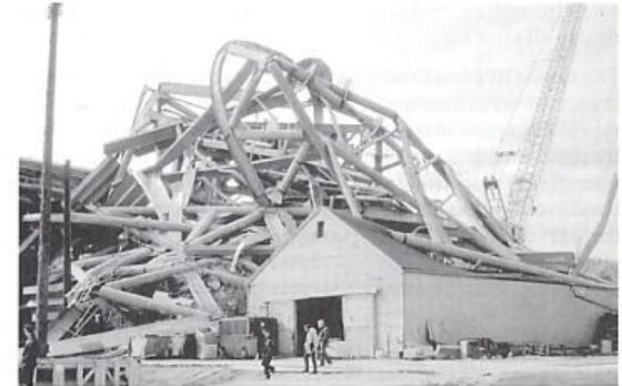
Figure 1.15 Stability and the strength of a structure—the collapse of a portion of the UW Husky stadium during construction (1987) due to a lack of adequate bracing to ensure stability. Photo by author.
