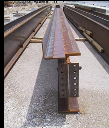
(AISC - Steel Structures of the Everyday)
