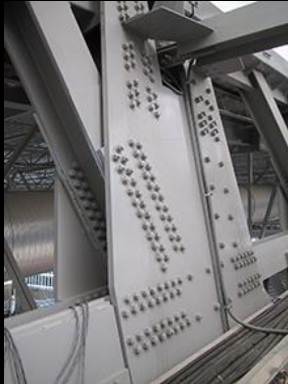
(AISC - Steel Structures of the Everyday)
