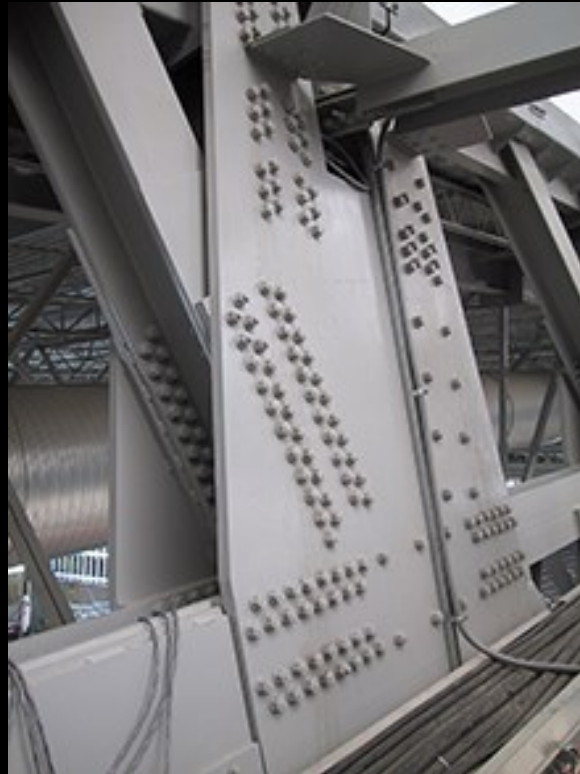
(AISC - Steel Structures of the Everyday)
