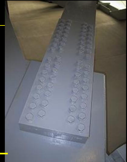
(AISC - Steel Structures of the Everyday)
