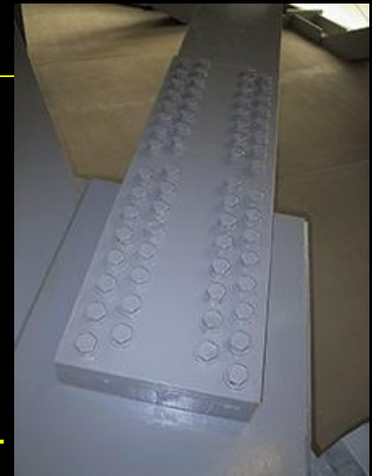
(AISC - Steel Structures of the Everyday)
