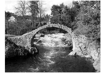
Packhorse Bridge, UK
